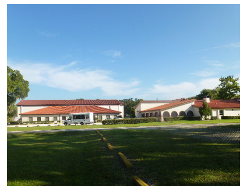
Safe and effective overflow parking areas.
